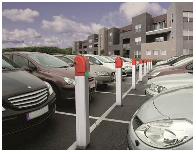
PHOTO 11. PARKING ELECTRIC PILLARS (PHOTO BY PRWEB)
